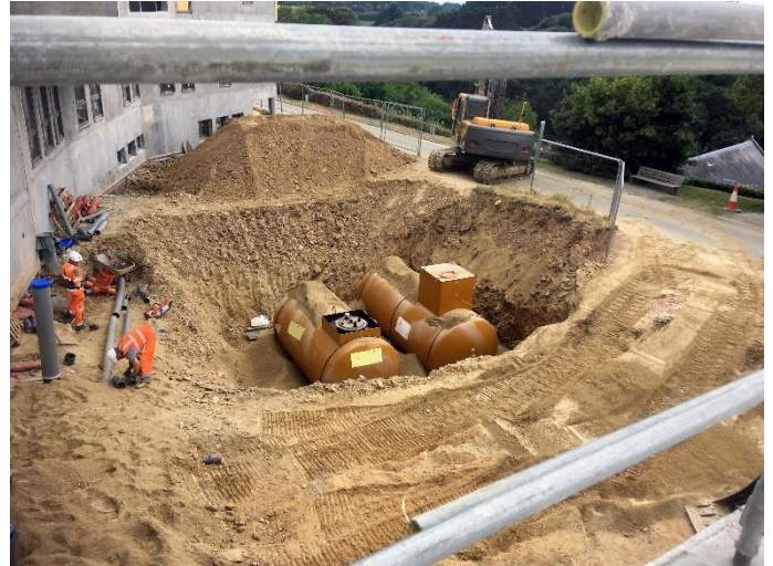
There are two underground tanks on the site: one for the generating sets and one for the fuel oil boiler room
