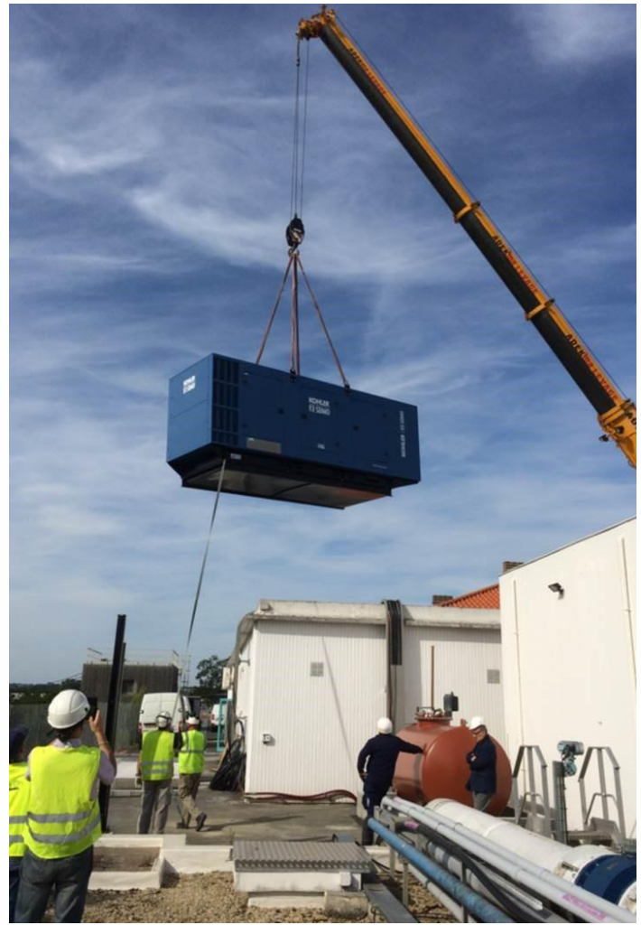
Pic. 4: The KD900 genset during installation on site
