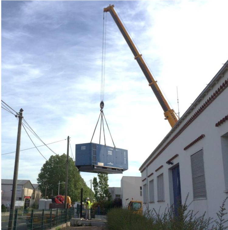
Pic. 3: The KD900 genset being lifted into position on site
